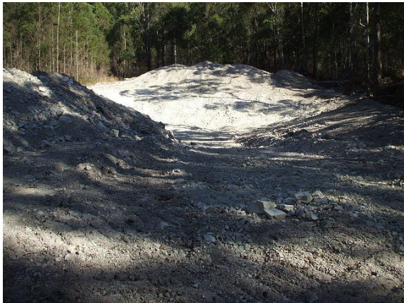
Localised excavation for extraction of access track materials within proposed residential development area
